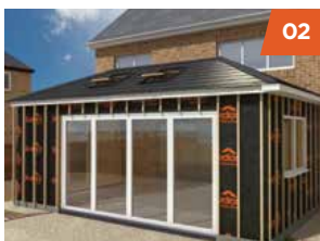
Timber battens are then secured to the outer.
