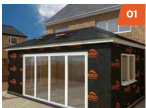
Breathable waterproof membrane is secured to the exterior walls.
