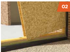
Wall and sole plates installed ready to receive the SIP panels.
