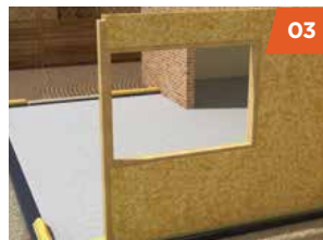
Subsequent panels are installed with specified window and door openings.
