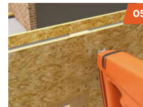
Wall panels are securely fixed together with a nail gun.
